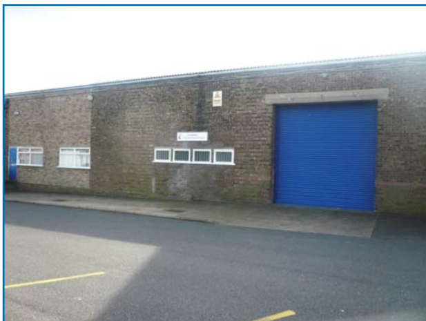
The immaculate unit K at the Kingsway Industrial Estate
